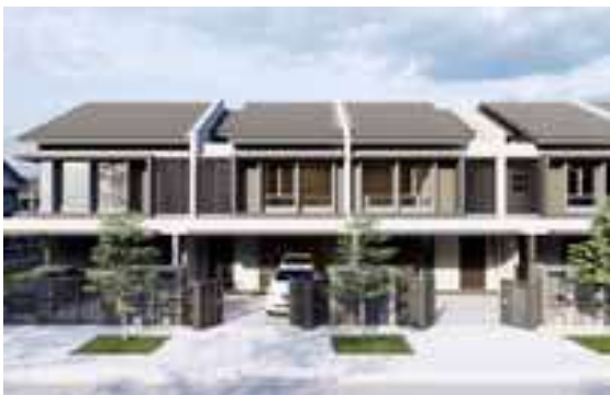
65 Units Double-Storey Terrace Houses
